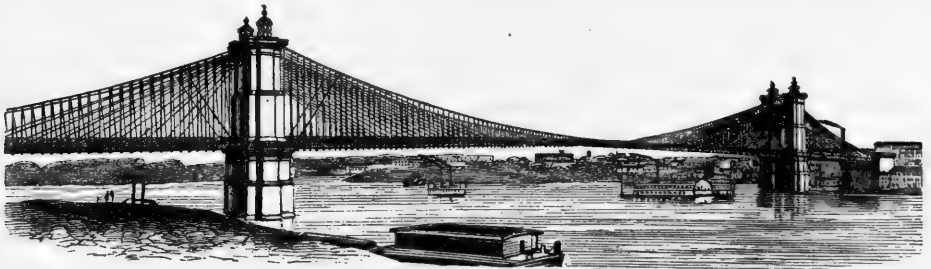
SUSPENSION BRIDGE OVER THE OHIO AT CINCINNATI.
